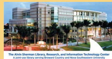
The Alvin Sherman Library, Research, and Information Technology Center A joint-use library serving Broward County and Nova Southeastern University
